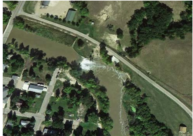
Lisbon Dam on the Sheyenne River in northeast Lisbon.
