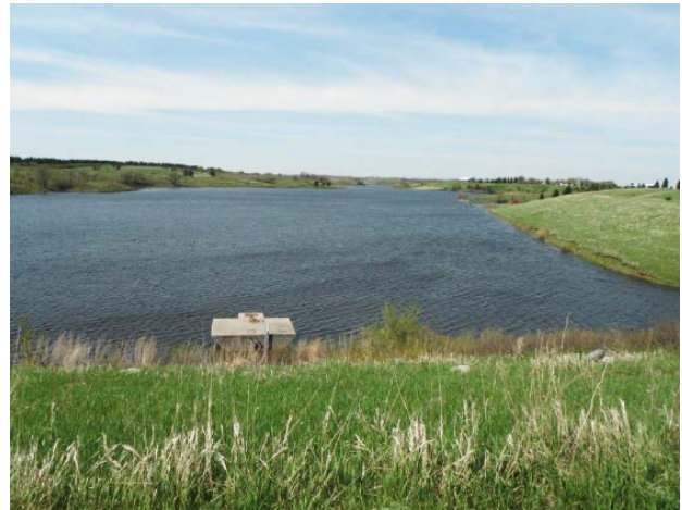
Dead Colt Creek Reservoir as seen from Dead Colt Creek Dam.
